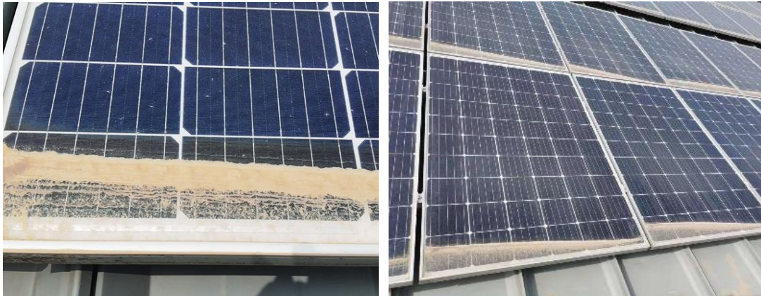
Dust is deposited at the bottom of the standard module
